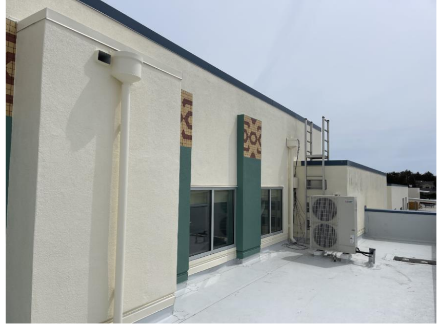
After (leaks repaired)
